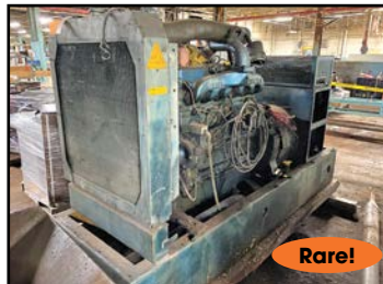
ALLIS-CHALMERS 110Kw DIESEL GENERATOR
